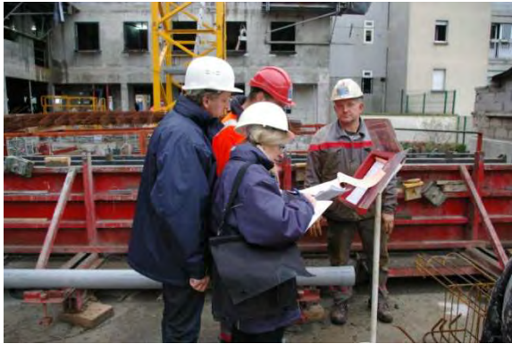
The Labour Inspectorate carrying out a check at a site in the Hauts-de-France Region © DIRECCTE Hauts-de-France Region
